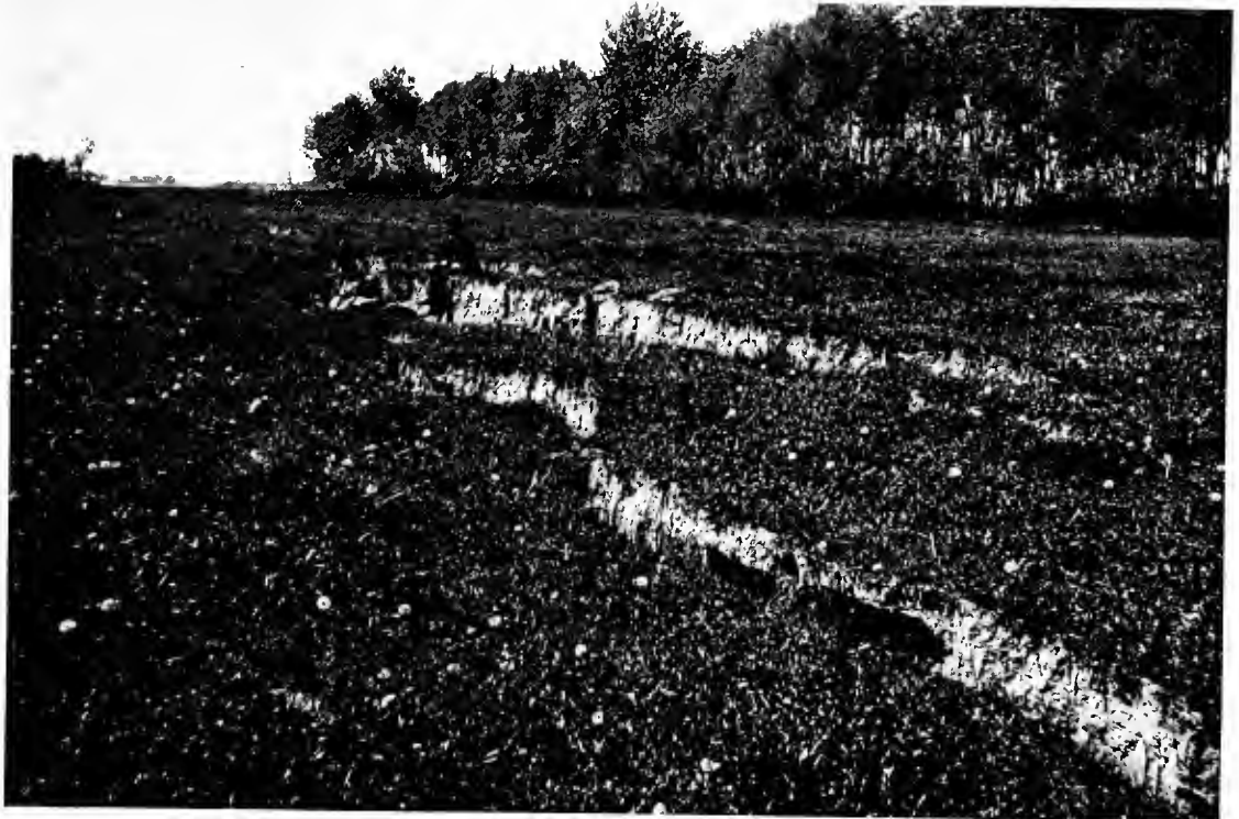
A. Eel River, near Ferndale. Cracks in flood-plain. A. S. E.
